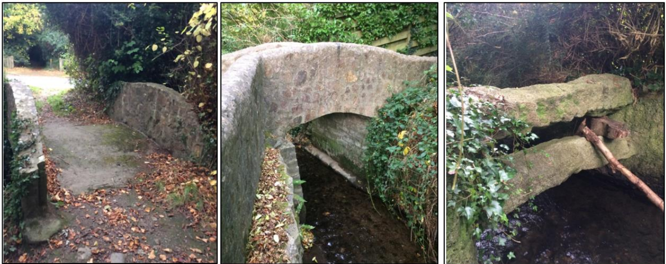
Figure 34 Bridges and foot bridge over the Three Trout River
