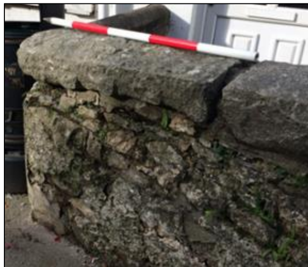
Figure 32 Granite capstone on the low rubble stone wall outside Beaumont Cottage, the underside of the capstone show evidence for stone cleave marks
