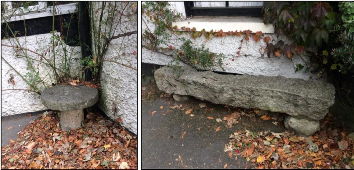
Figure 33 Mushroom stone and reused granite pier outside the Long House, cleave marks are identifiable on the pier
