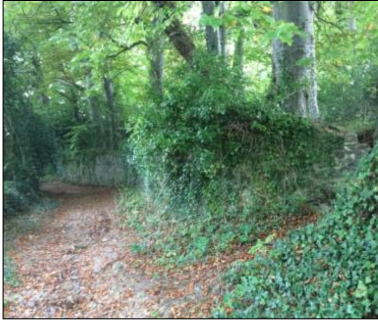
Figure 35 Rubble stone walls aligning Blackberry Lane
