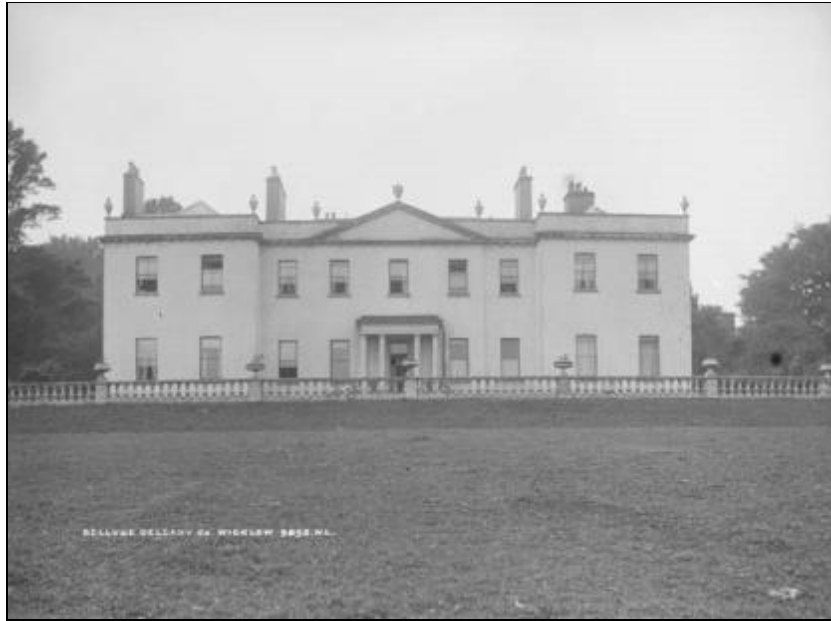
Figure 17 View of Bellevue Laurence Photograph Collection [between ca. 1865-1914].
